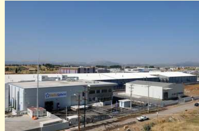
Production Facility, Tripoli Greece
