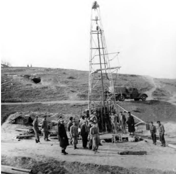
75. The artesian well drill in Damiano Giannitsa (March 1952).
