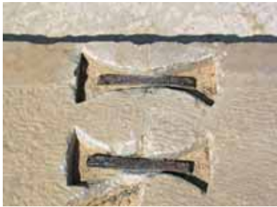
Fig. 5 Pasargadae. 'Dove-tail' clamps. Takht-e Jamshīd Library Archive.
