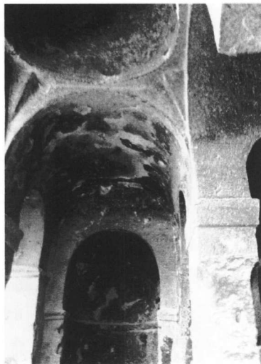
Fig. 16. Yaprakhisar Area 10, church A. General view of interior, looking east
