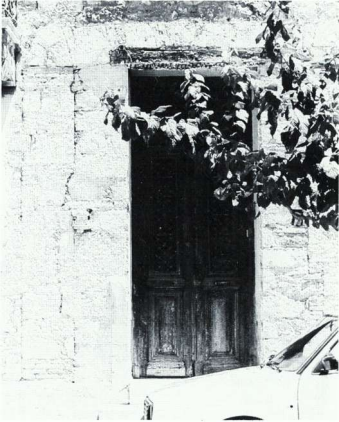
18. Recent photograph of the entrance to one of the houses, showing the adaptation of the opening.
